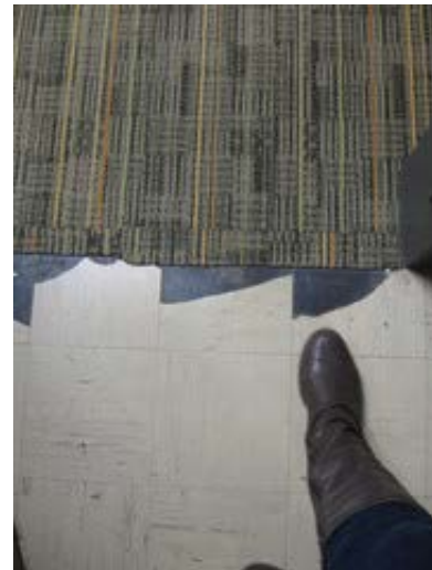
Hallway with Damaged Tile
