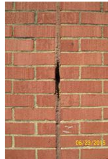
Control Joint to be Caulked
