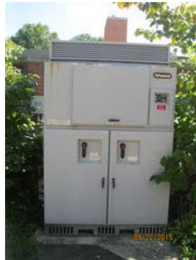
Solar Power Inverter/Switchgear
