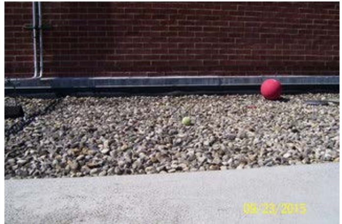
Typical Ballasted EPDM
