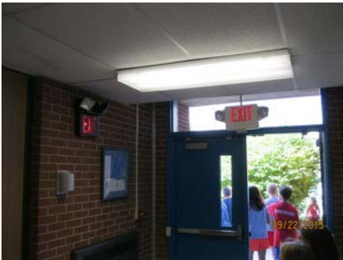
Door Security Contacts/Exit Signs/FA Pull Stations
