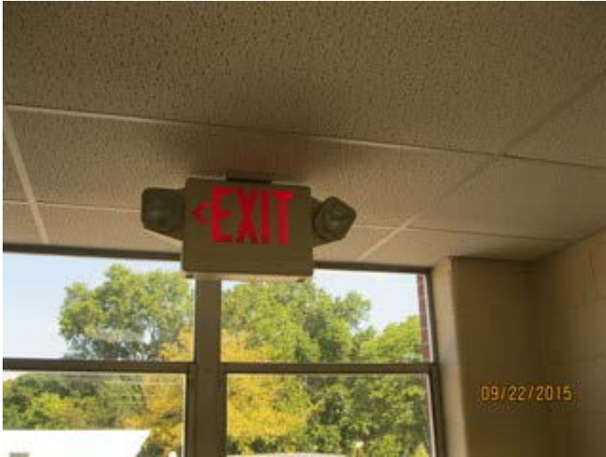
Exit Sign With Remote Heads
