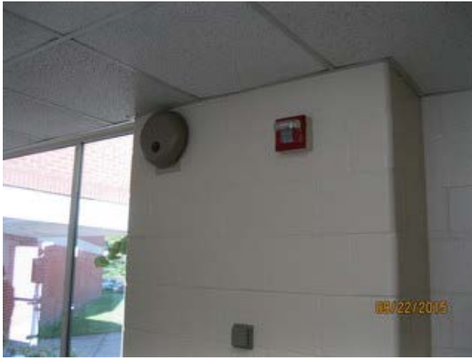
Fire Alarm Horn Strobe
